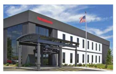
Eave / Rake Extensions and Canopies Canopies and overhangs are available to enhance the exterior appearance of your building. Canopies and eave/rake extensions offer a great aesthetic as well as functional option. The following designs are most commonly used:
