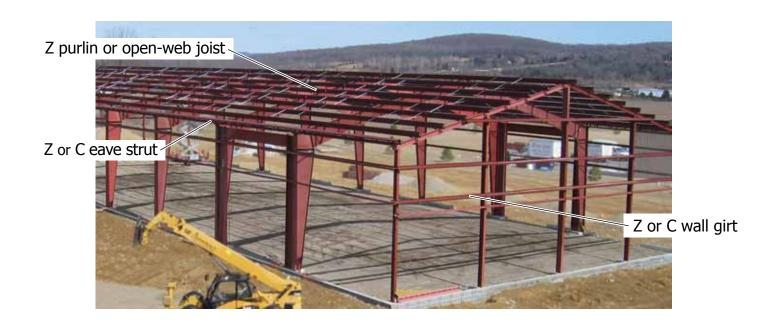
Wall Structurals Nucor Building Systems provides 8", 10", & 12" sidewall girts depending on wind loading and column spacing. Sidewall girts can be designed for either inset or bypass applications. Bypass girts offer the most economical sidewall design and are practical when walls are partially open for masonry.
